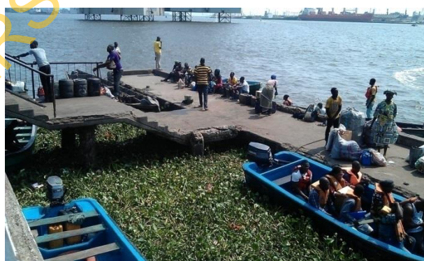
Plate 3: Poor facility of Jetty (CMS) in Lagos Island
