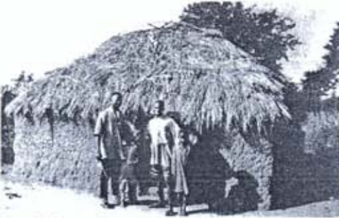
Plate 1: Farm house of mud wall and thatch roof
