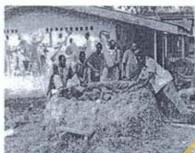
Figure 1: Dried termite mound bricks being set for burning in a mud-kiln Figure 2: Veneers and iron rods used to mark the circular foundation
