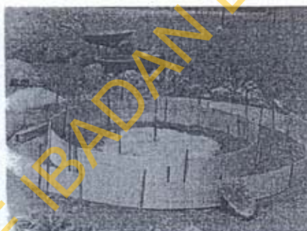
Figure 1: Dried termite mound bricks being set for burning in a mud-kiln Figure 2: Veneers and iron rods used to mark the circular foundation
