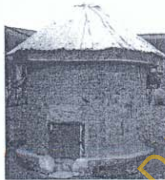
Figure 7: Completed silo showing the manhole to which the discharge chute is attached
