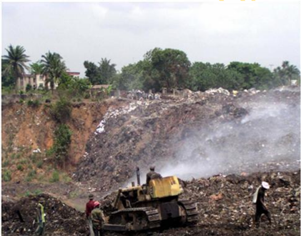
Figure 2.2: A typical dumpsite (Unsanitary landfill) in Nigeria without landfill liners, covers and leachate collection systems. It is located in proximity to residential quarters, with regular burning of wastes.
