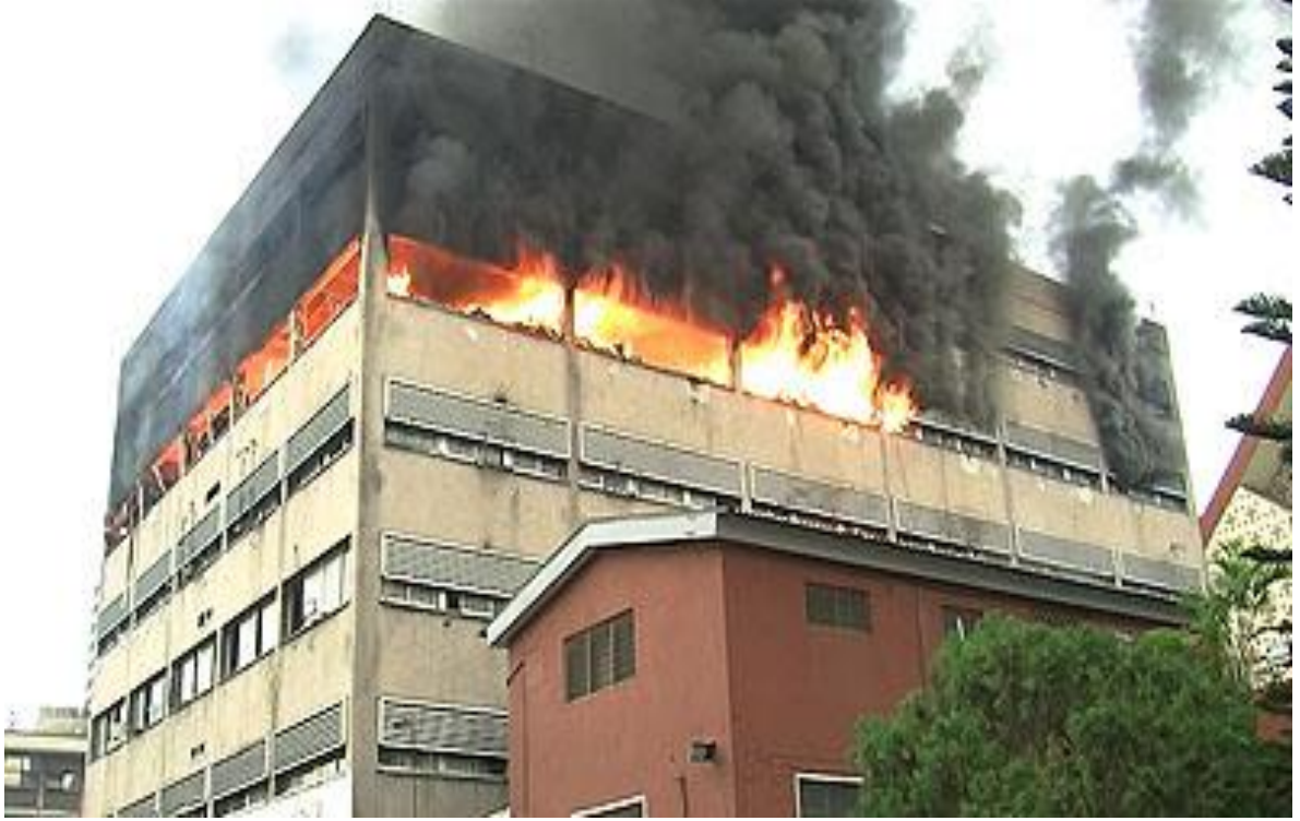
Plate 7.2 Fire disaster at Euroasia Plaza, 10/12 Breadfruit Street, Lagos
