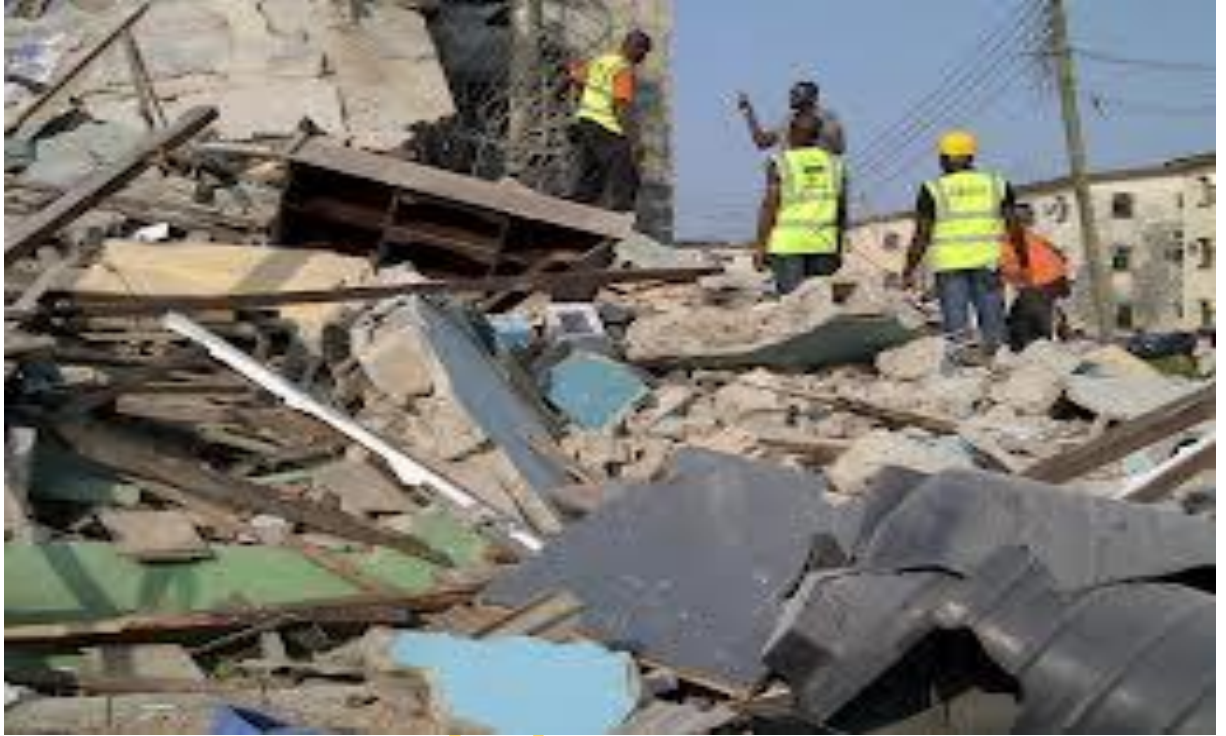
Plate 7.4 Collapsed residential building at Jakande Estate, Oke Afa, Oshodi Isolo, LGA.
