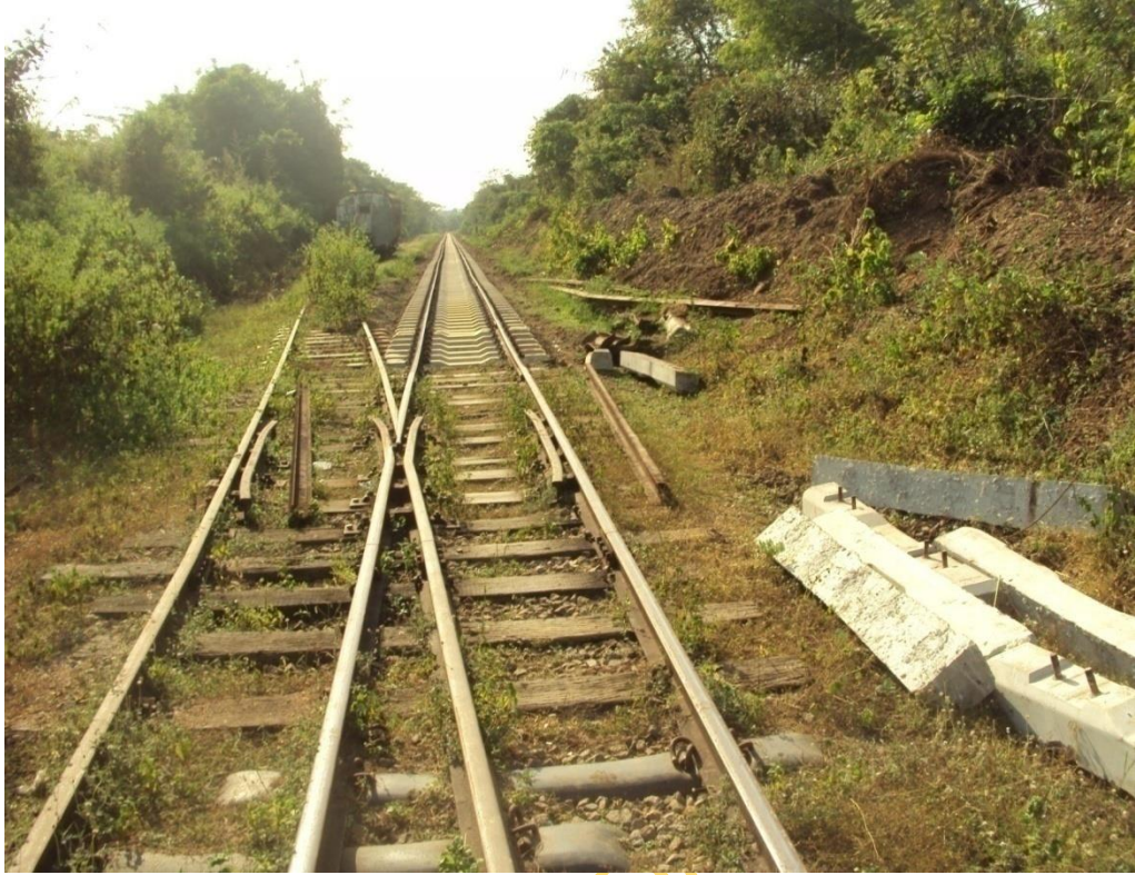
Plate 4.1: On-going Repair Works on the Old Rail Tracks Source: Field Survey, 2011
