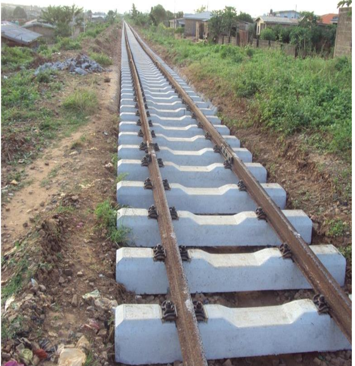
Plate 6.1: The New-Look Concrete Rail-Tracking in Ibadan.
