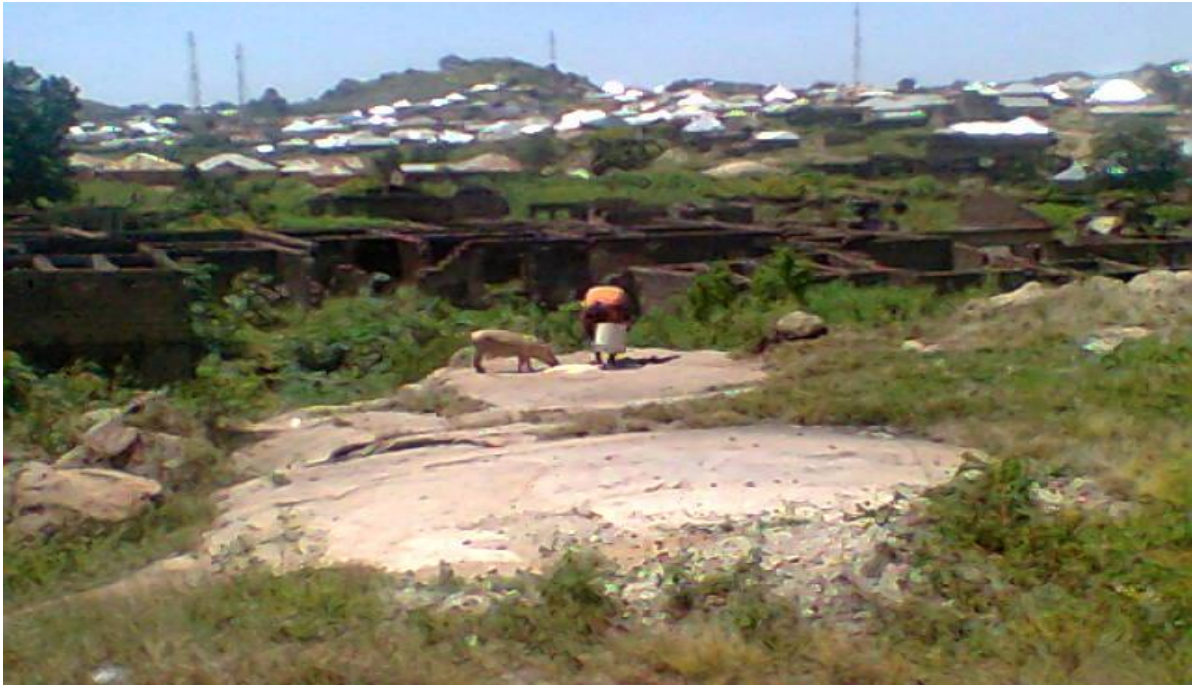
Destroyed buildings between Rikkos and Jos Jarawa
