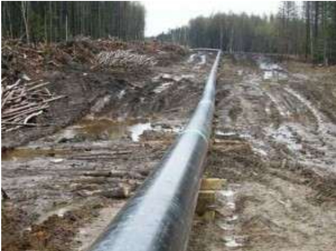
Fig. 1.12: Pictures showing some replaced vandalized pipeline at baruwa
