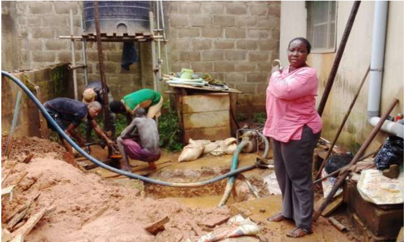
Fig. 3.4: Drilling of borehole to collect sample at different intervals
