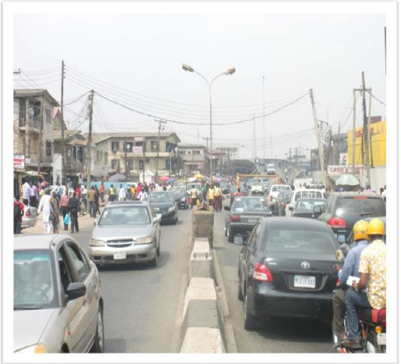
Plate 6.2: A roadway in Ikeja with a divide but Lack Buffer and Walkways
