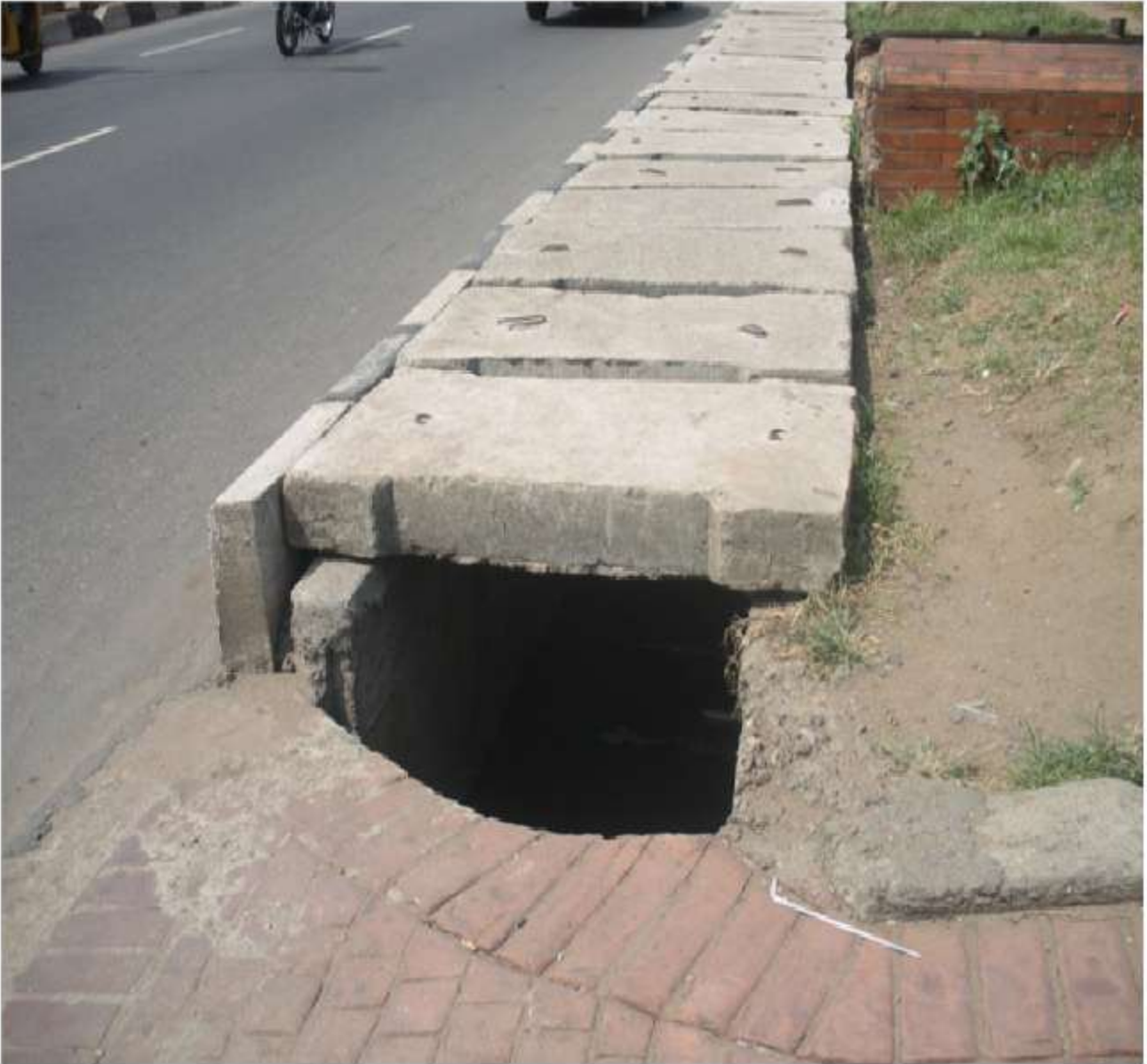
Plate 4.6: Covered Drainage Used for Pedestrian Walkway along Lateef Jakande Road.
