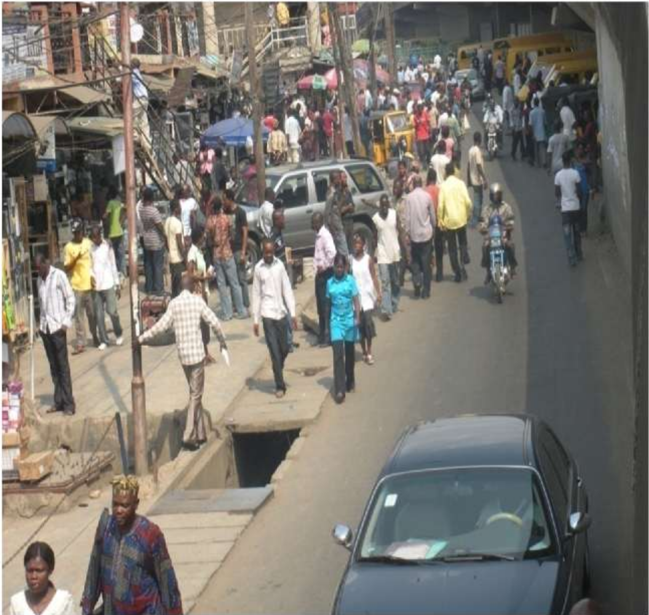
Plate 4.7: Pedestrians Avoiding Uncovered Drainage Used as Walkway along Obajaland Kodesoh Street.
