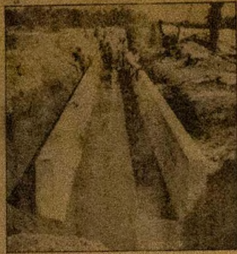
DESIGN UNDER CONSTRUCTION AT OBALENDE FOLLOWING LAND FILLING
