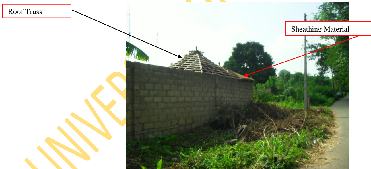
Plate 2.1: Roof Assembly Showing Truss and Sheathing
