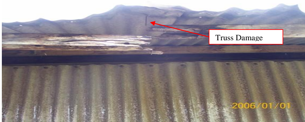
Plate 4.6: Truss Damage
