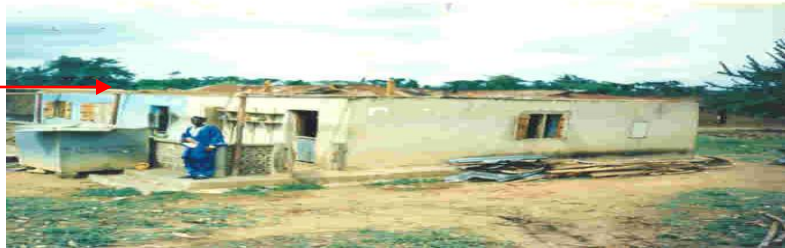
Plate 4.1: Roof Blown-off
