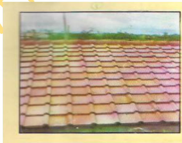
Plate 2.5b: Roof constructed with Tile
