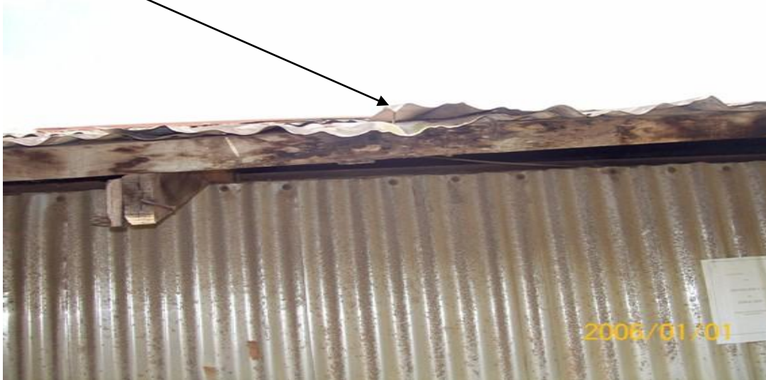
Plate 4.3: Nail Withdrawal
