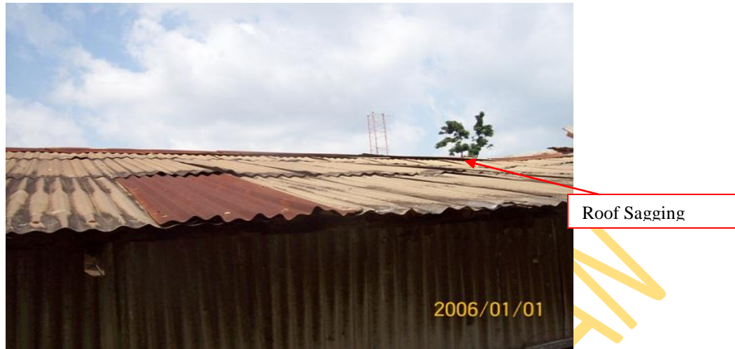
Plate 4.10: Roof Sagging
