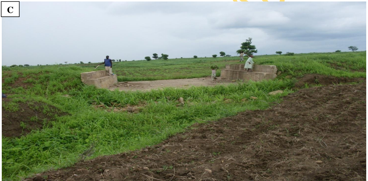
Fig 4.14; Babam dam failure
