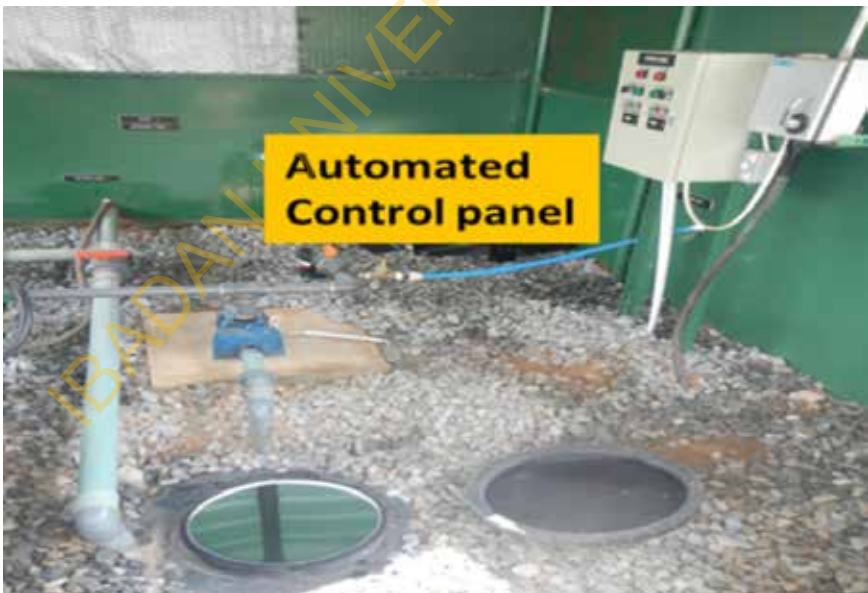
Figure 20. Power house showing an opened 1000-L tank with the nutrient pumping pipe.
