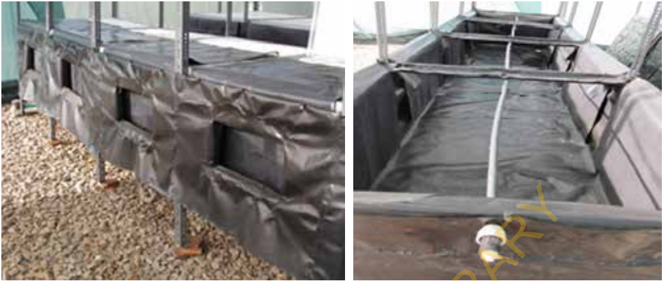
Figure 12. Styrofoam fully covered with black plastic sheet outside the box (left) and inside (right).
