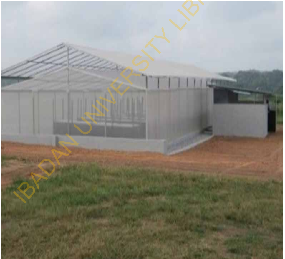
Figure 16. Fully completed power house adjacent to the aeroponics screenhouse.
