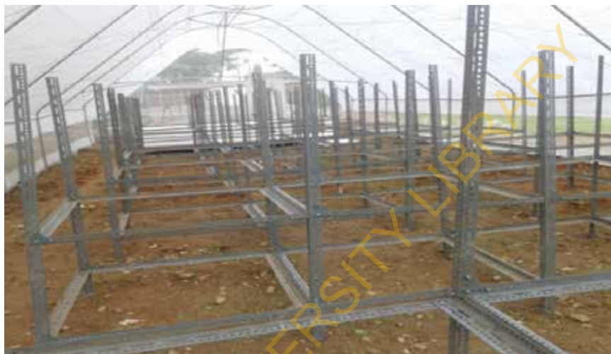
Figure 9. Construction of the aeroponics boxes frames using Dexion shelf.
