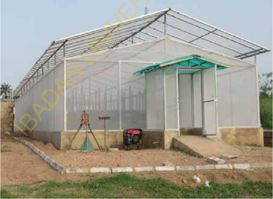
Figure 7. Global view of completed aeroponics screen house with double ceilings.
