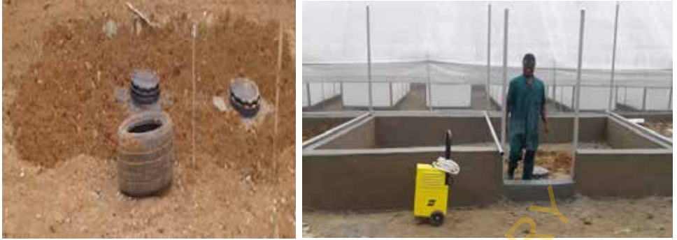
Figure 15. Left picture are tanks of 1000 l buried and right is the mason work of the power house.
