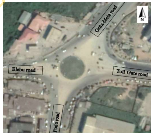
Plate 2: Aerial view of New Garage Roundabout Source: [10]
