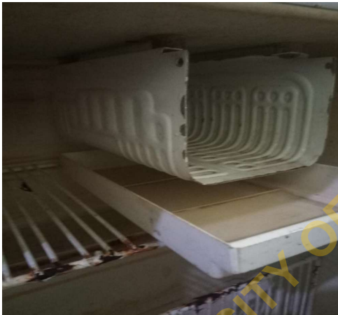
Fig 2: A picture of the Evaporator in the refrigerator
