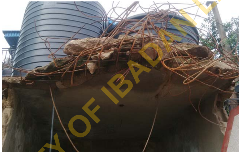
Plate 3. Showing the Partial Demolition State of Case 2
