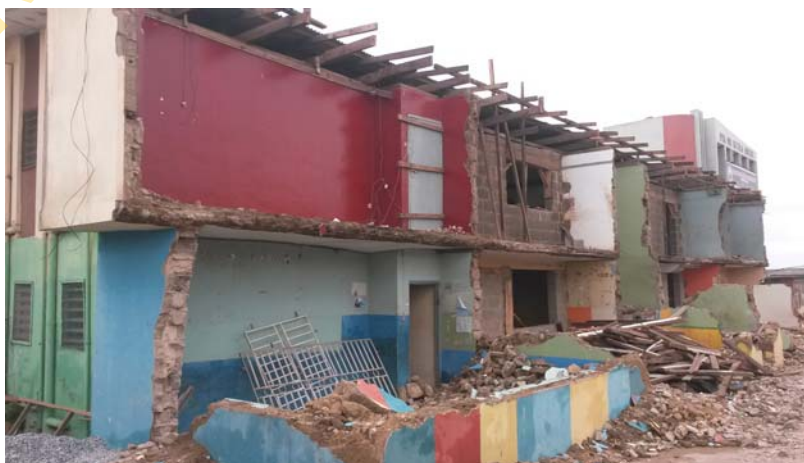
Plate 2. Showing the Partial Demolition State of Case 1
