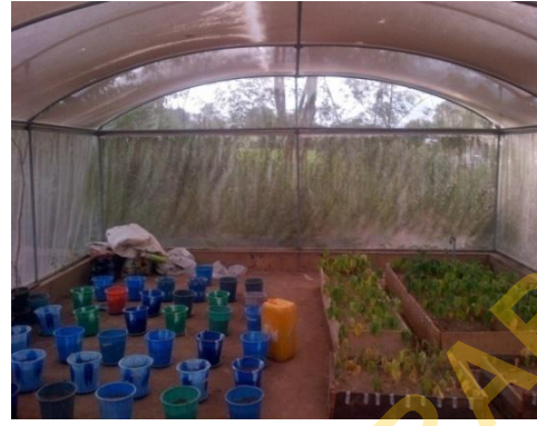
Plate 9: Dust Accumulation on Roof and Screen.
