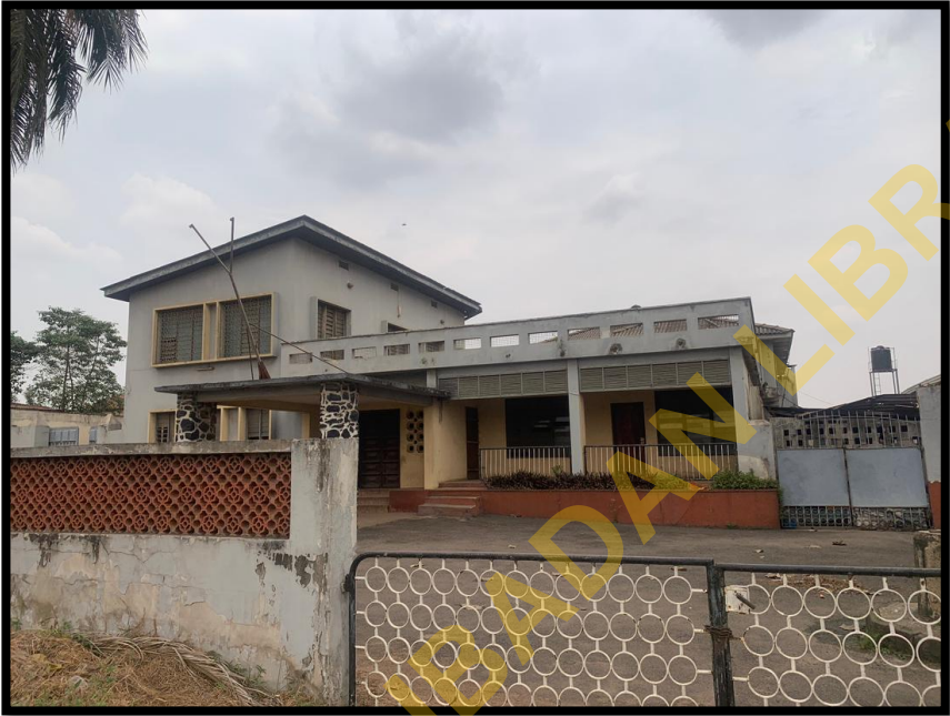
Figure 3.9: Obafemi Awolowo House, Dugbe: Fieldwork (2022)
