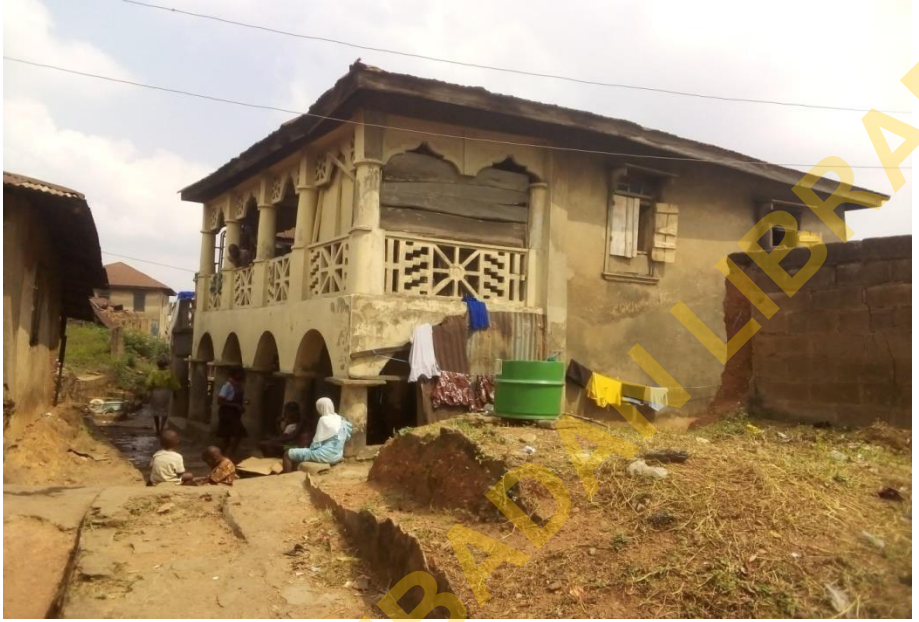
Figure 5.9: A storey building with 5 rooms at Beere. Source: Fieldwork 2022
