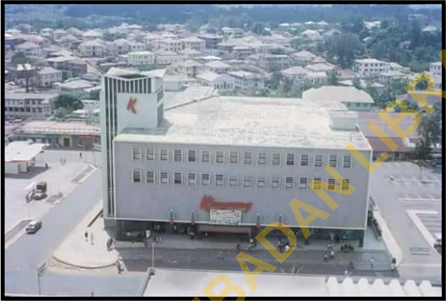
Figure 3.7: Old Kingsway Building. Source: Fieldwork (2022)
