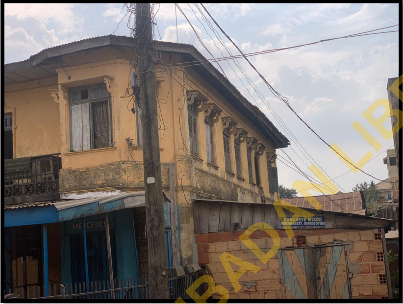
Figure 4.1: An old residential apartment under study.
