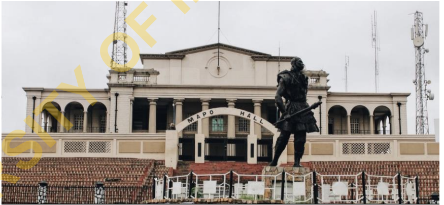
Figure 5.16: Entrance to Mapo Hall: Fieldwork 2022
